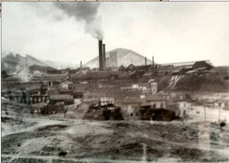
Cananea Consolidated Copper Company, 1906
